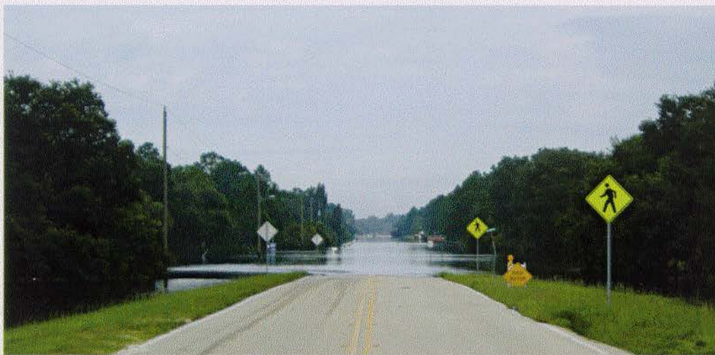
Figure 5 —View of road overflow at discharge of 4,450 ft 3 /s, Big Slough Canal at Tropicaire Boulevard near North Port (site 8, fig. 1, table 1) on June 24, 2003.
