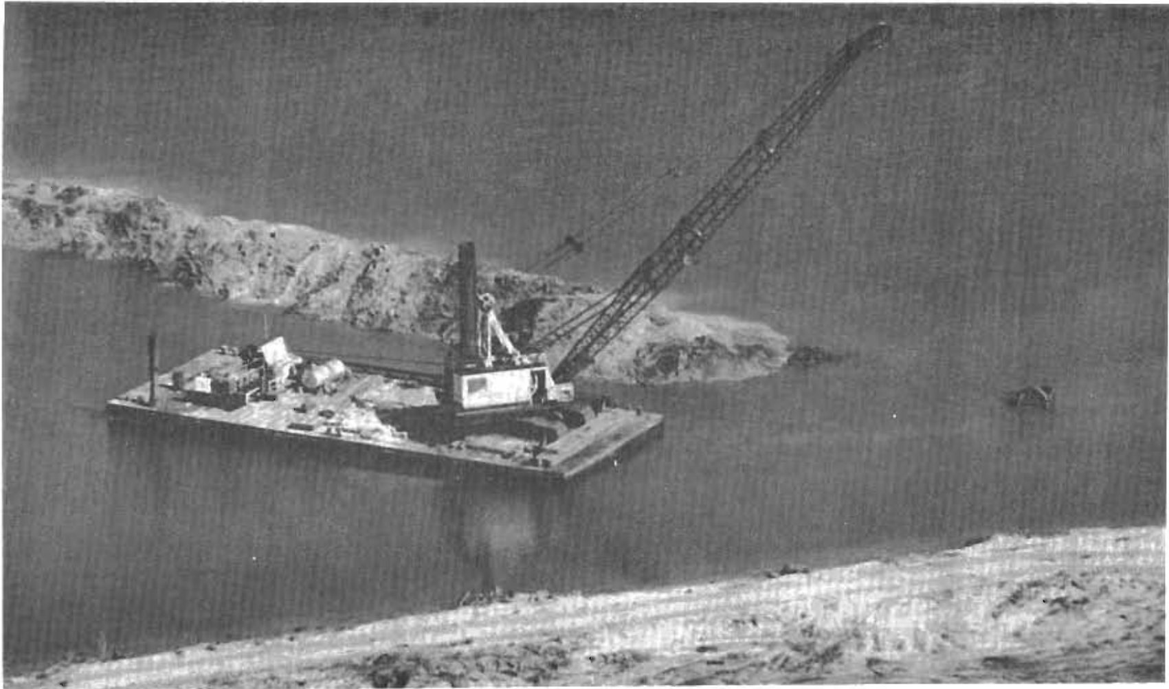
Figure 3. Port Manatee Construction, 1969. Dragline building phase dike adjacent to cleared shoreline. Dredged material will be pumped behind dike to extend land seaward.
