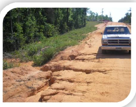
This picture shows the erosion caused by stormwater overtopping the unpaved road. Sediment is washed into the stream.
