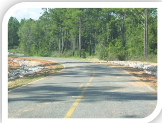
The picture to the right shows the completed section of Trout Toad, fully stabilized. The 6% slopes in the parallel swales are rep-rapped to prevent washout.
