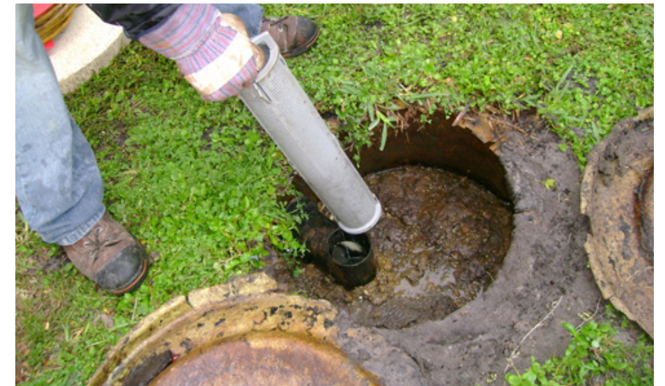
The US. Environmental Protection Agency recommends that septic tanks be inspected every three years and pumped out every 3–5 years.
