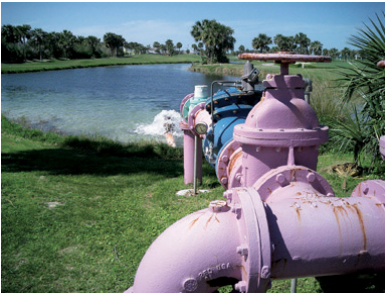
Reclaimed water pipes are painted purple for easy identification.
