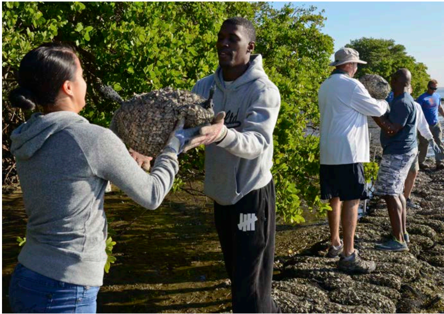
Volunteers helped install bags of oysters along the shoreline at MacDill Air Force Base to reduce erosion and provide habitat. Photos courtesy of MacDill AFB.
