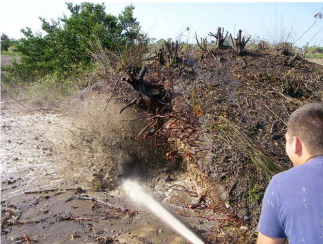
Hydroblasting with high-pressure water hoses is an efficient technique for removing spoil mounds from wetlands that were historically ditched and drained for mosquito control. Photo courtesy of SWFWMD.
