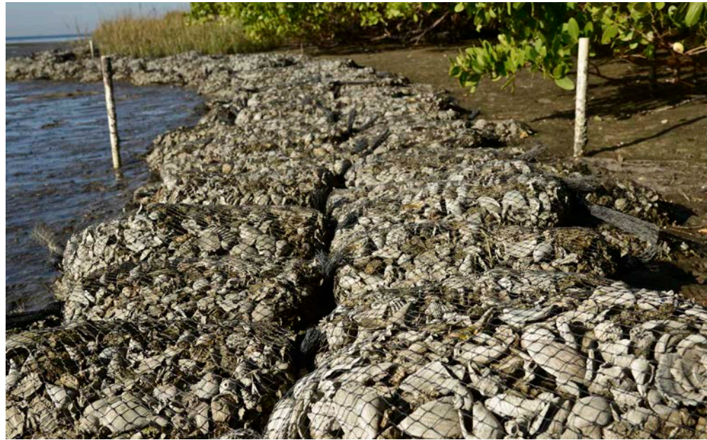
Volunteers helped install bags of oysters along the shoreline at MacDill Air Force Base to reduce erosion and provide habitat. Photos courtesy of MacDill AFB.
