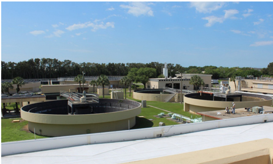
St. Petersburg’s Southwest WWTP is producing fertilizer from bio-solids and fuel from bio-gas generated by the treatment process.
